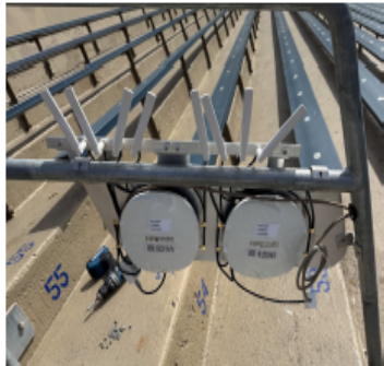
(b) APs mounted on a handrail.
