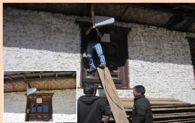
Before and after (inset) the installation of the Television White Space antenna and base station at a health center in Tang, Bhutan.
