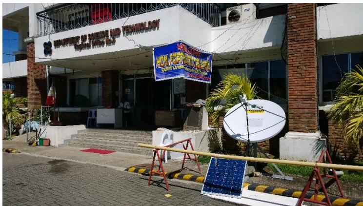
DOST Region 8 Office (with VSAT and solar panel) where the base station was located.
